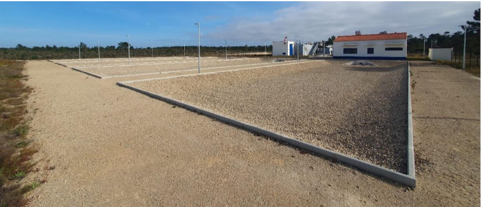
Infiltration basins at Comporta wastewater treatment plant managed by Águas do Alentejo SA (AgdA) (photo: Marcel Horovitz)
